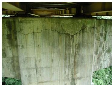
Fig. 6 Example of a bridge deteriorated by ASR
