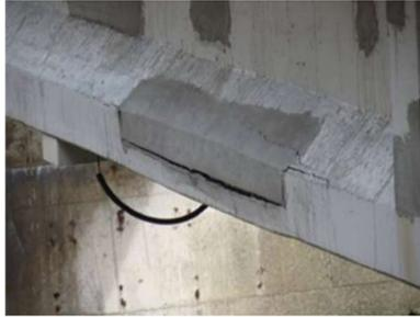
Fig. 7 Example of re-deterioration due to macrocell corrosion after patch repair
