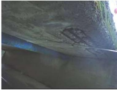
Fig. 4 Short-span bridges where superstructure concrete has fallen due to initial defect
