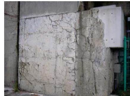
Abutment of a viaduct damaged by ASR
